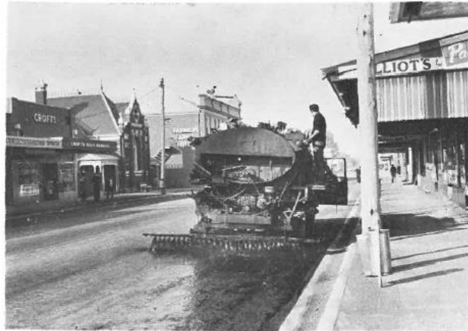
SEALING NEWLY CURBED MELVILLE STREET IN 1966. A. J. Pumpa, Photo
