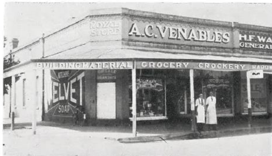
THE ROYAL STORE, which was converted from Royal Mail Hotel on enr. of Saxton and Melville Streets.
