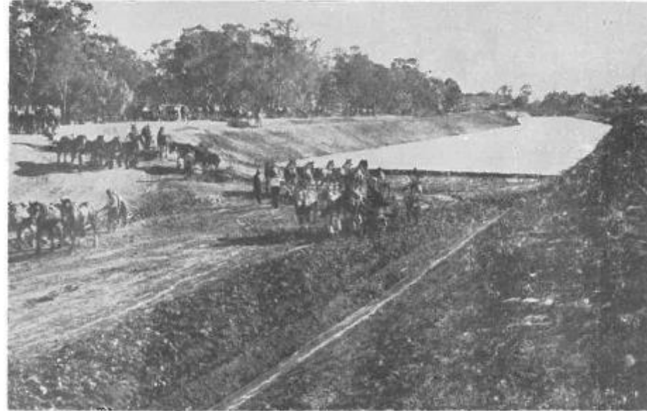
OVER 100 HORSES WERE USED IN CONSTRUCTION OF MAIN CHANNEL IN IRRIGATION WORKS FOR SOLDIER SETTLEMENT NEAR NUMURKAH.
