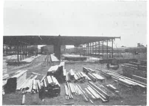
TECHNICAL WING UNDER CONSTRUCTION
